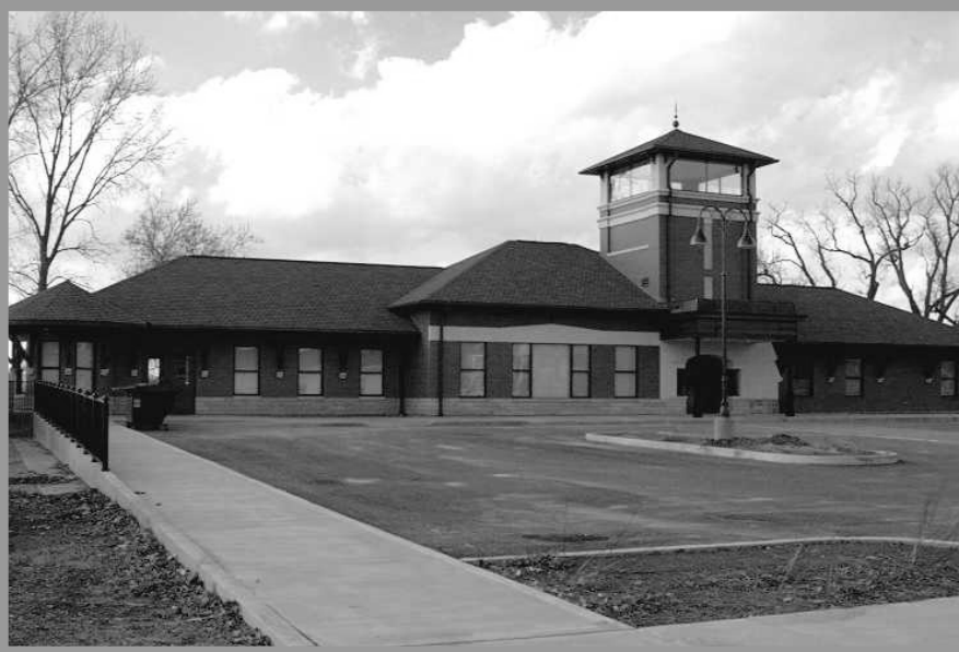
This nearly completed Welcome Center on the river front in Henderson, KY is a near replica of the old L&N passenger depot which will probably not be restored. It's a shame to lose the old building but this structure will be an excellent reminder of past railroad grandeur. digital image by
